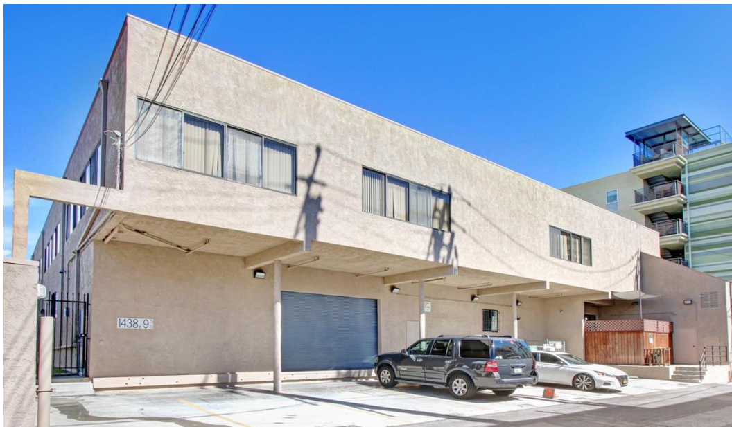
Real Alley Access Loading
